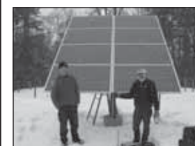
Owner John Blittersdorf and helper install a solar panel
