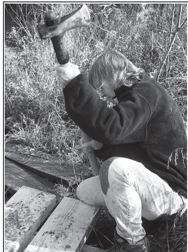
Barbara Griffith works on building a footbridge on the Long Trail.
