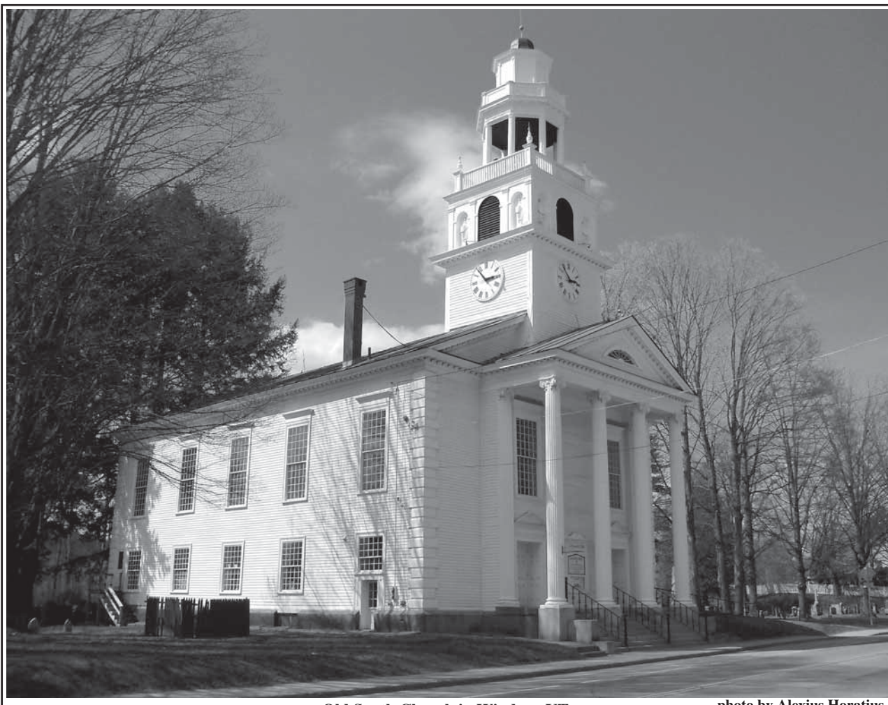
Old South Church in Windsor, VT.
