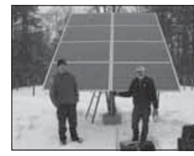
Owner John Blittersdorf and helper install a solar panel
