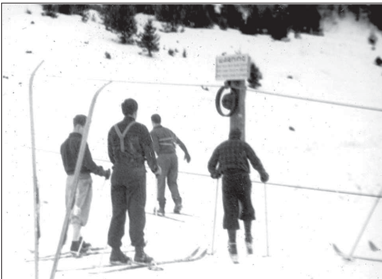
photo courtesy of Woodstock Historical Society Skiing via rope tow in early Vermont. The first ski lift in the Eastern United States, an improvised rope tow powered by a Ford Model T engine, was installed at Suicide Six ski resort in South Pomfret, VT in January 1934.
