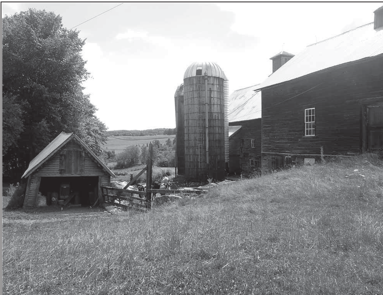
An old wood-stave silo at the Allen Butler farm in East Montpelier, VT. photo by Claude Stone
