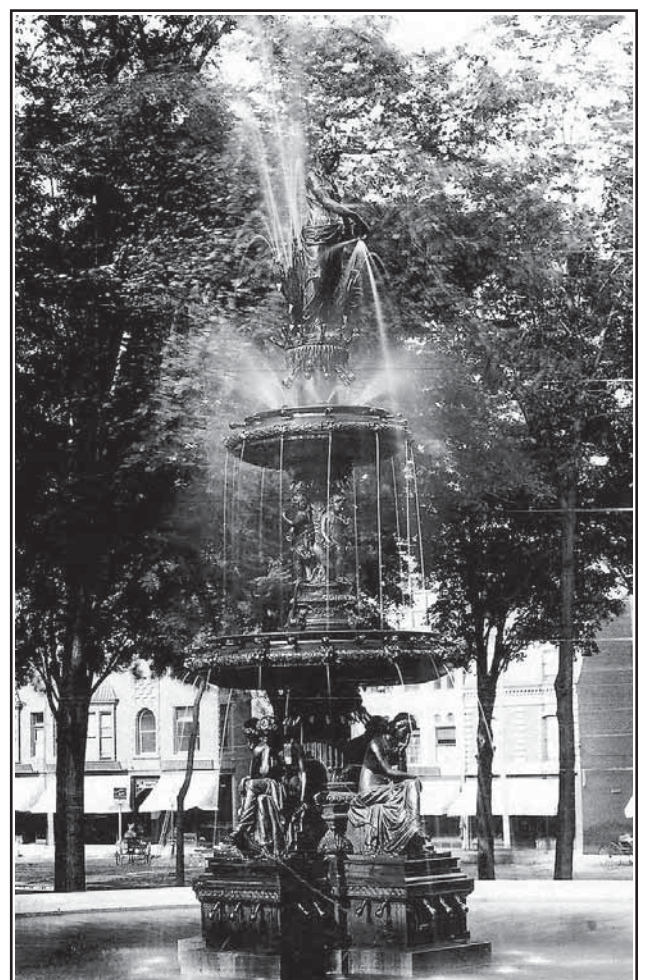
The restored fountain in Taylor Park, St. Albans, VT.
