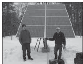
Owner John Blittersdorf and helper install a solar panel
