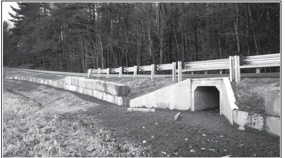
The town of Monkton recently completed this highway project that allows amphibians to pass under the road unharmed. This location previously risked thousands of amphibian deaths in a single night.
