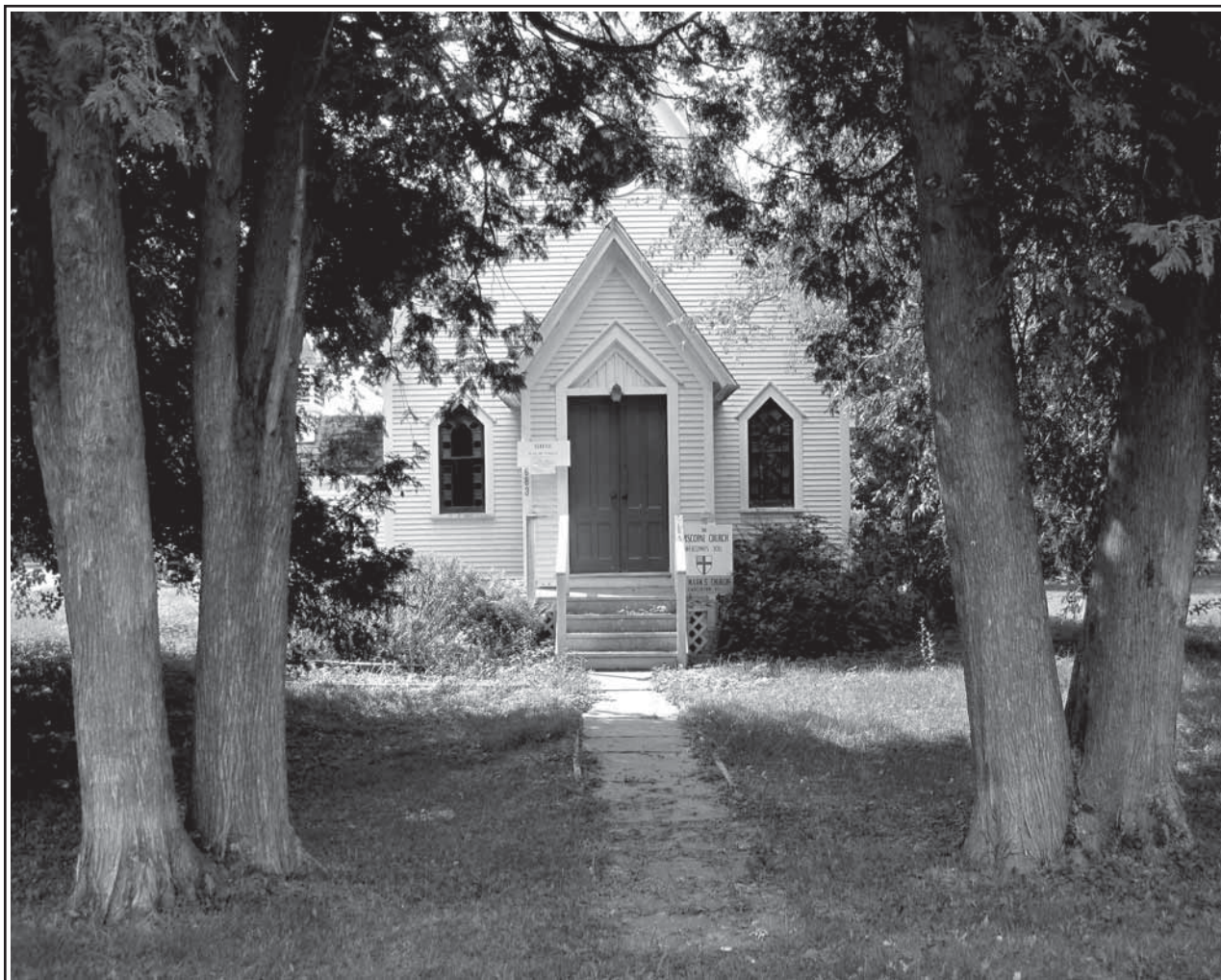
The former St. Mark's Church in Castleton, VT.
