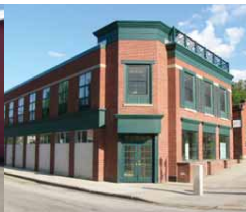
2 SOUTH MAIN STREET 10,000 SQUARE FEET
